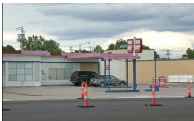
Abandoned service station sites present many issues for future use.
