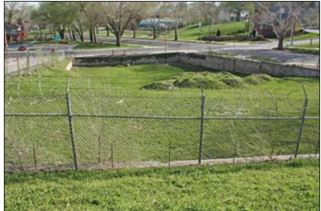
Sites of former manufacturing facilities, such as this former Kansas City thermometer manufacturing site, may pose hazards for future use.
